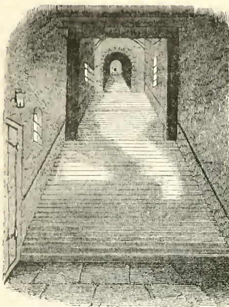
STAIRCASE TO THE ROUND TOWER.
